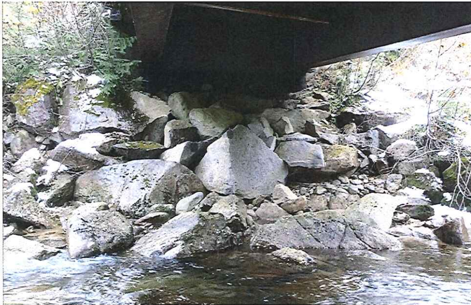
CK2316 Left Abutment
