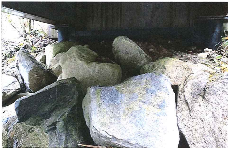
CK2316 Right Abutment
